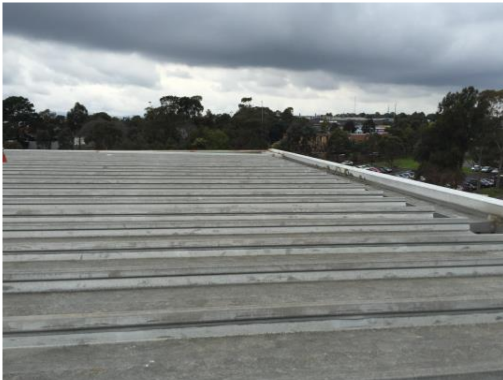
Site Photograph 22 – very slight fall in fly tower roof deck
