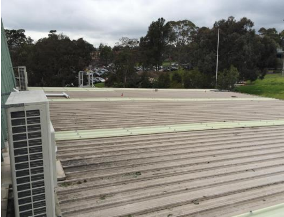
Site Photograph 13 – main roof areas had a number of anchor points
