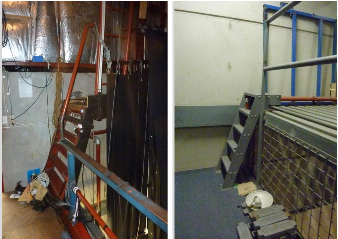
Figure 8: Loading gallery handrail mesh safety measures from other venues
