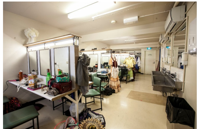
Dressing Room 1 – insufficient dressing rooms leads to different users having to share inappropriately – especially children
